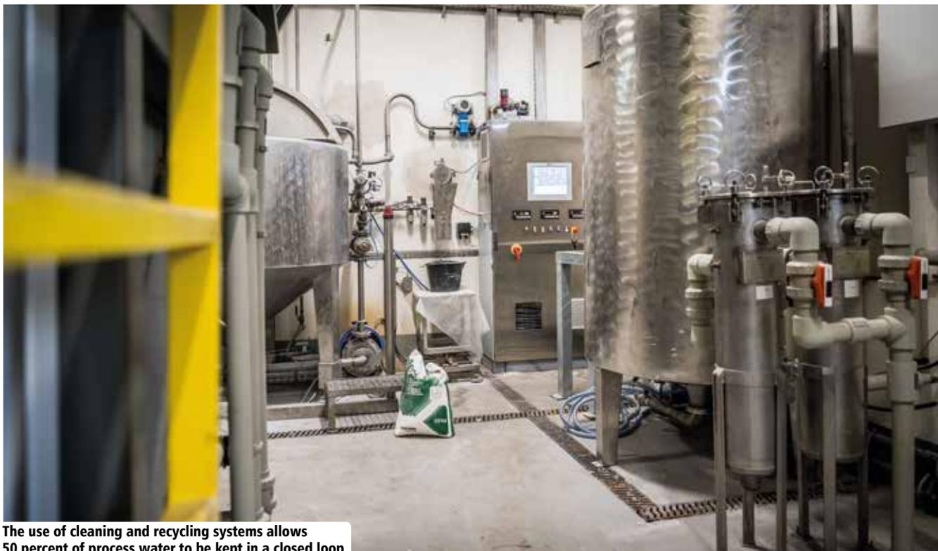
**The use of cleaning and recycling systems allows 50 percent of process water to be kept in a closed loop**
